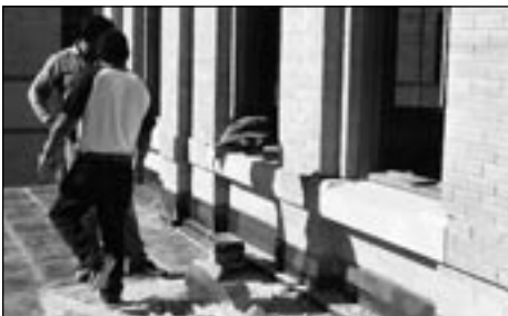
Limestone window sills were replaced.
